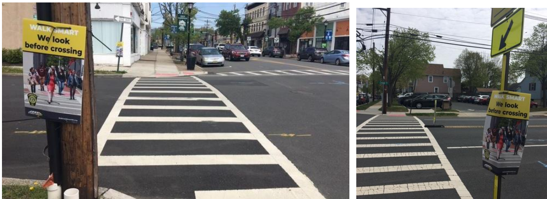
Figure 13a and b: Street Smart Signs Near Post Office, One Block from Focus Intersection
