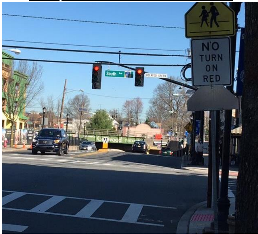
View of rail bridge near the train station
