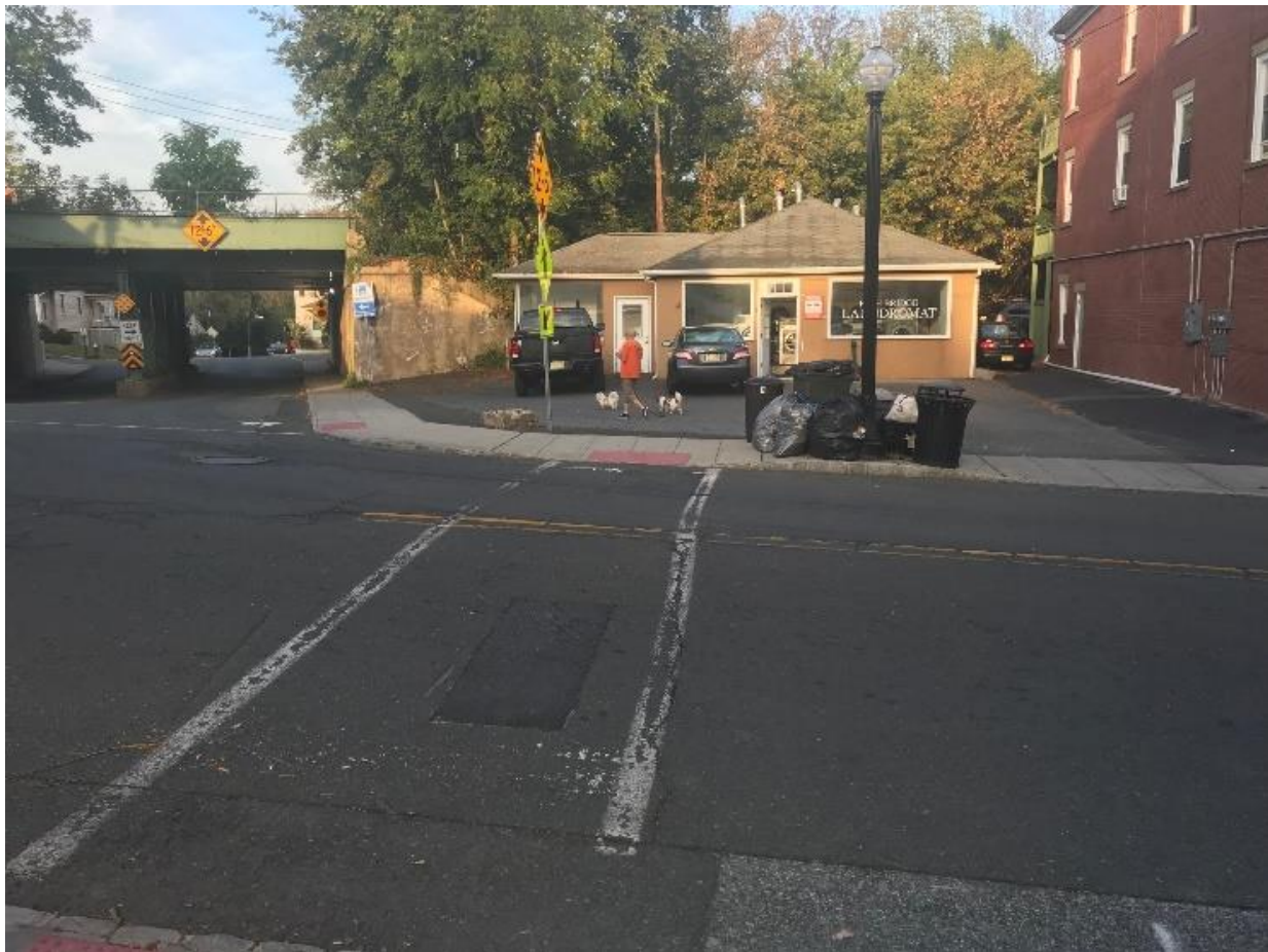
Before: Main Street Crosswalk
