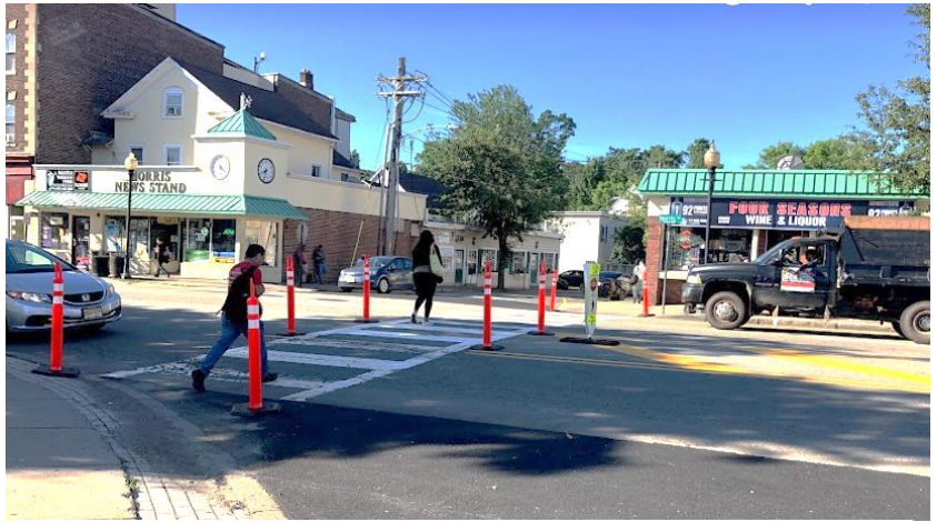
Temporary Delineators at Intersection of Morris Street and King Street
