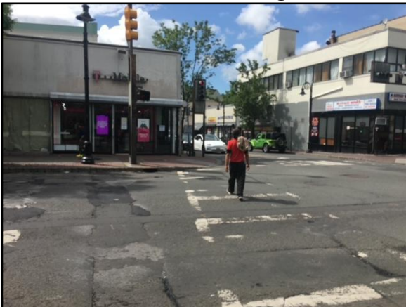
Crosswalk is not fully painted
