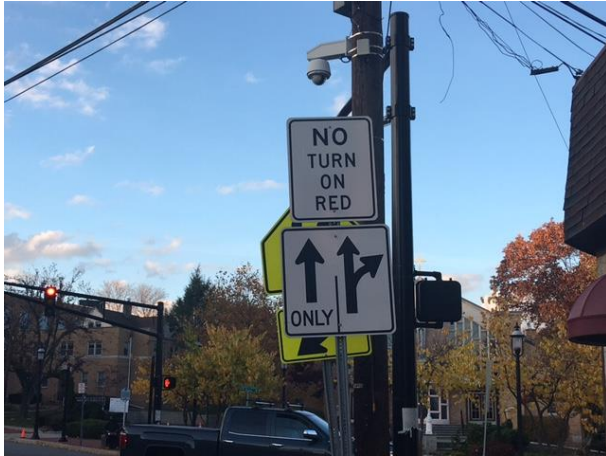
Fig. 8a: No Turn on Red Sign Obstructs Ped Sign
