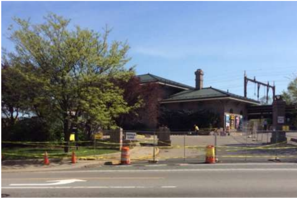
CONTRUCTION AT MORRISTOWN TRAIN STATION – MAY 12, 2016
