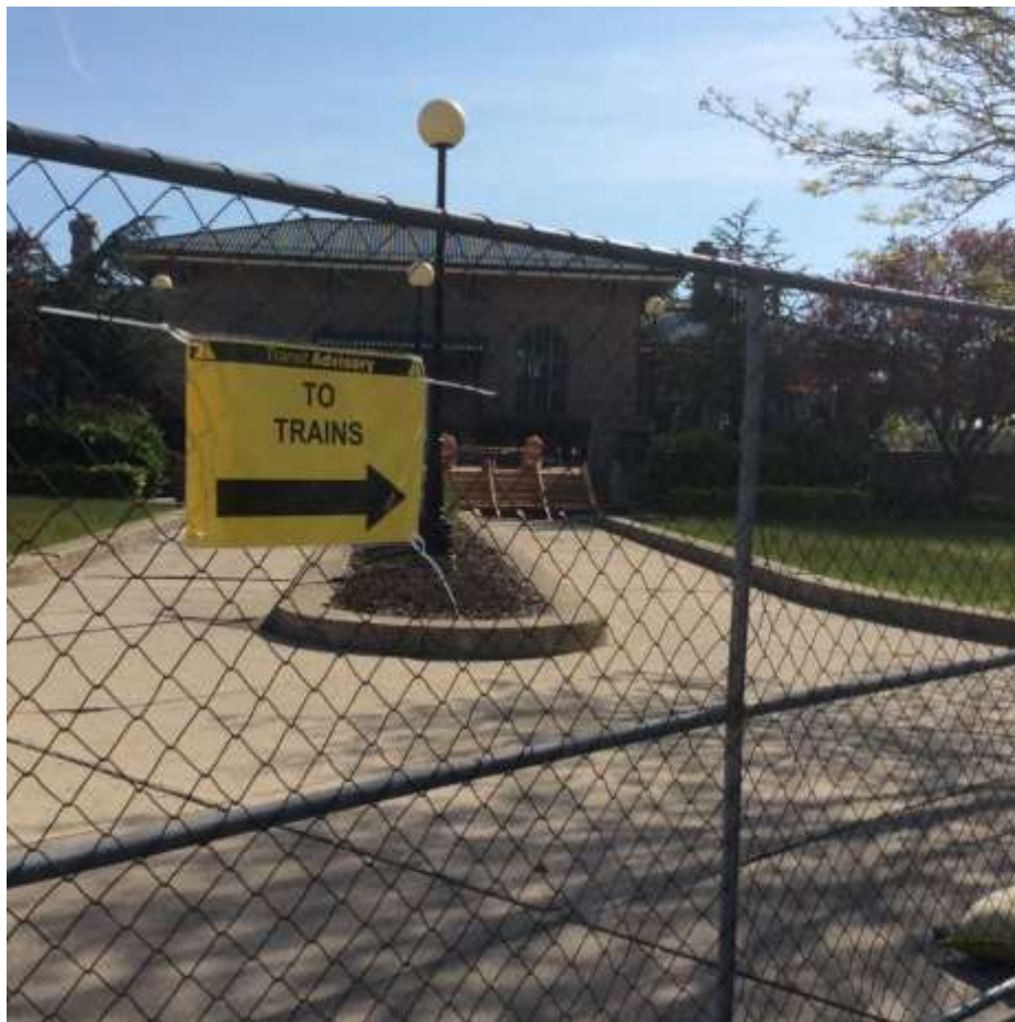
CONTRUCTION AT MORRISTOWN TRAIN STATION – MAY 12, 2016
