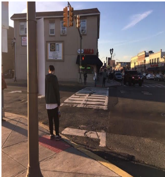
Crosswalk is Not Fully Painted
